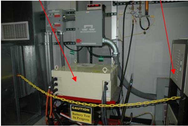
Figure 2(b).The JCS Battery with the power, communication and the coolant connections.
